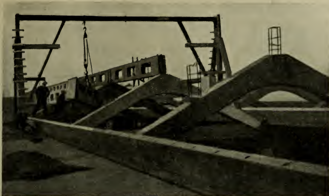
NEW WORKSHOPS FOR THE GAS LIGHT & COKE CO.: HOISTING PRE-CAST CONCRETE PURLINS INTO POSITION.
